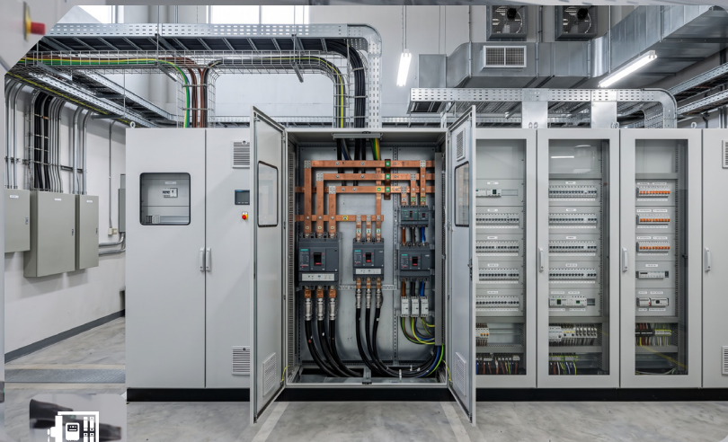
● Electrical Distribution Board (DB / SDB / MDB)
