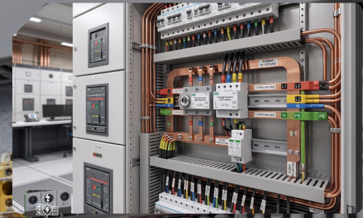
● Surge Protection Systems (SPD)
