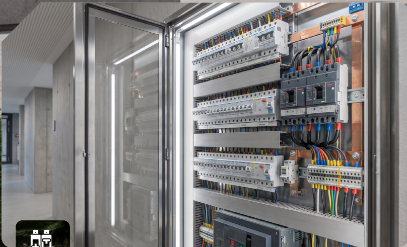
● Circuit Breakers (MCB / MCCB / RCCB / ACB)
